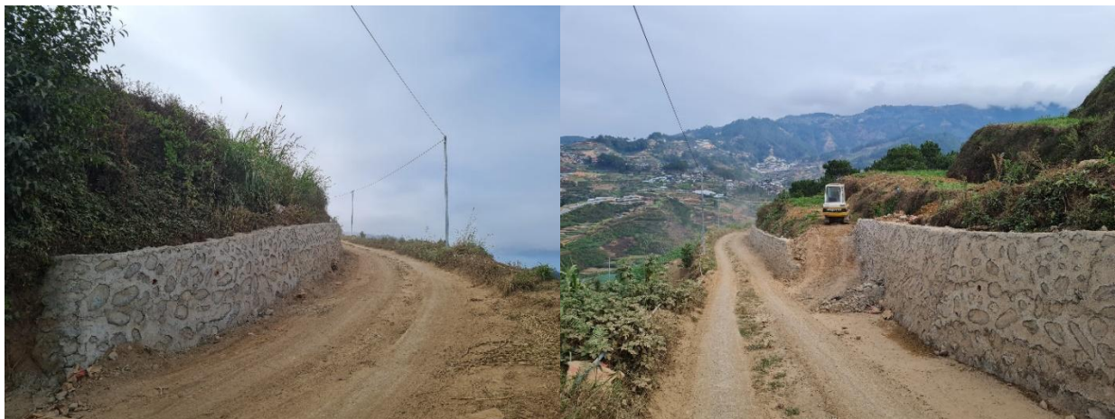
Photo 5. Riprap extension towards CDH-61 drill site.
