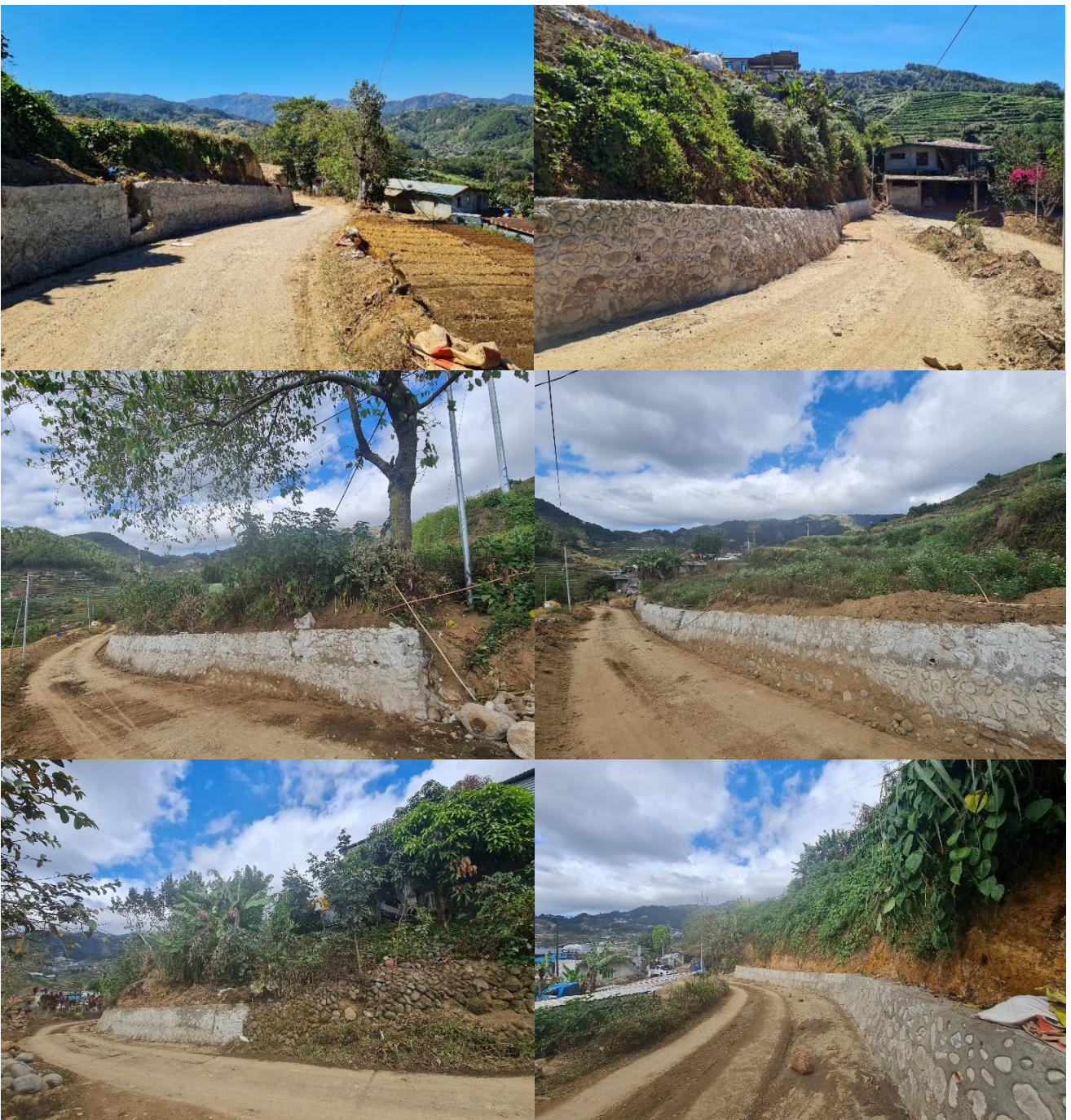
Photo 8. Riprapping and excavation works going downhill to Sitio Colocol.
