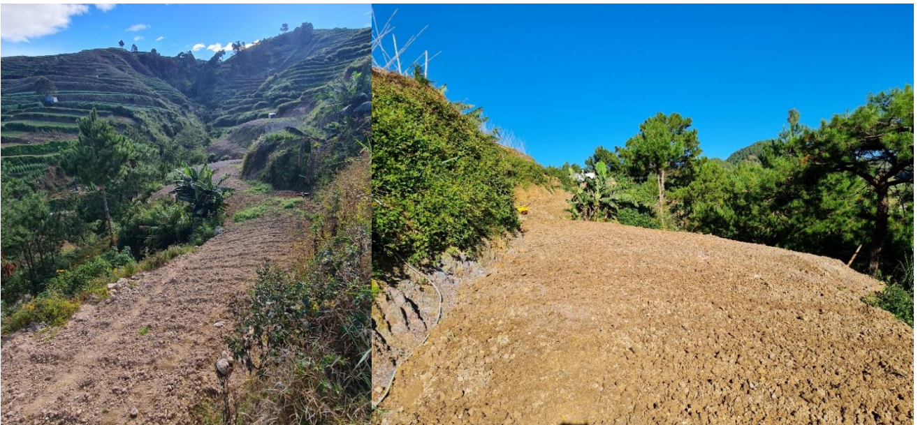
Photo 2. CDH-62A drill platform as of February 12, 2023.
