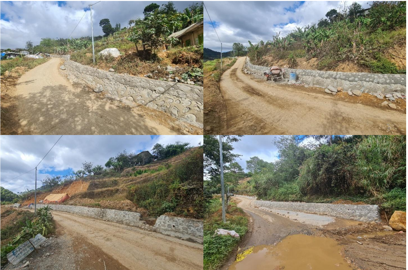
Photo 10. Riprapping excavation works from Maggangan creek going uphill to Sitio Colocol.
