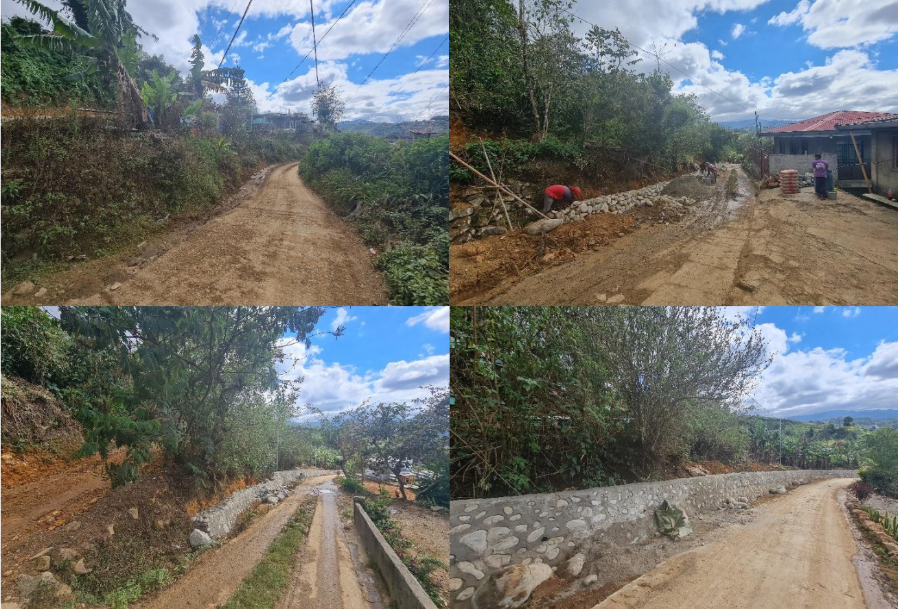
Photo 9. Riprapping and excavation works going downhill from Sitio Colocol going to Maggangan creek.
