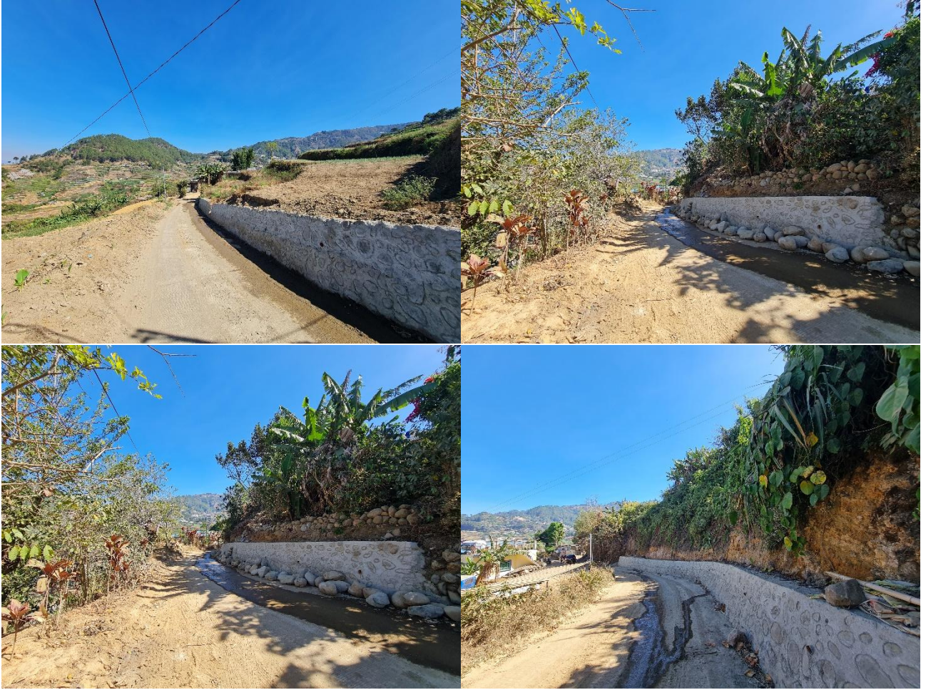
Photo 4. Riprapping going downhill to Sitio Colocol.
