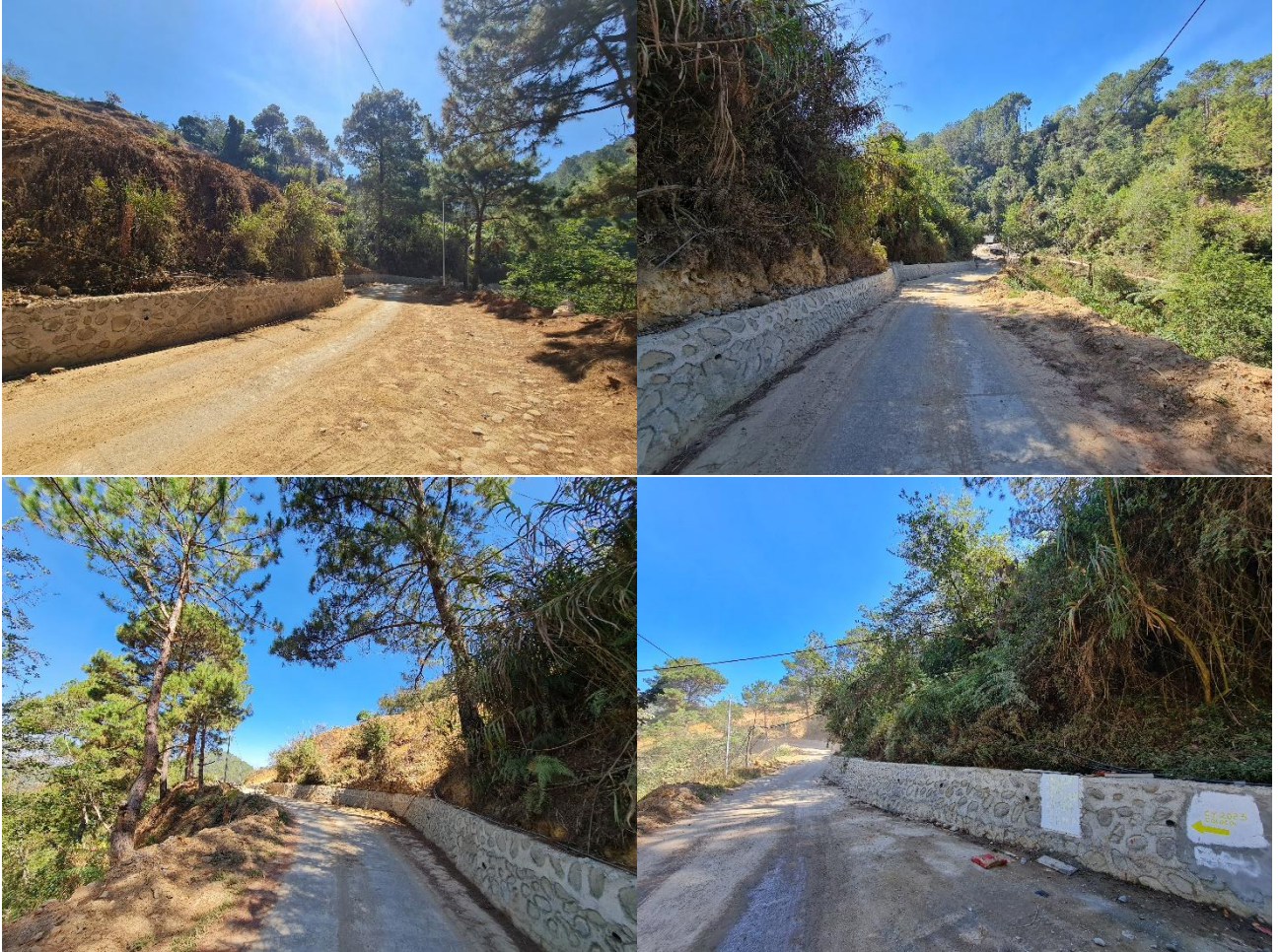
Photo 6. Riprapping going downhill from Sitio Colocol going to Maggangan creek.
