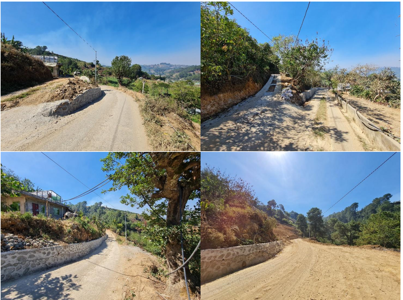
Photo 5. Riprapping going downhill from Sitio Colocol going to Maggangan creek.
