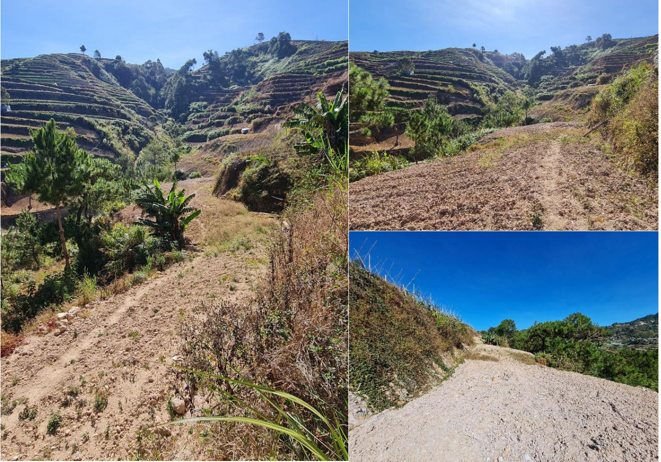
Photo 2. CDH-62A Drill site rehabilitation as of March 24, 2023.
