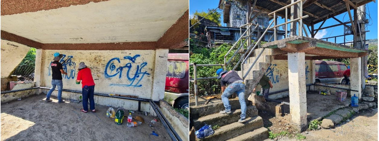
Photo 1. Rehabilitation of waiting shed.
