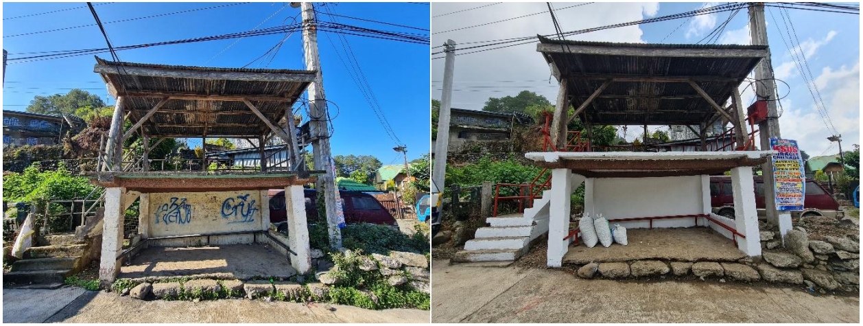
Photo 3. Before and after photos of the rehabilitated waiting shed.
