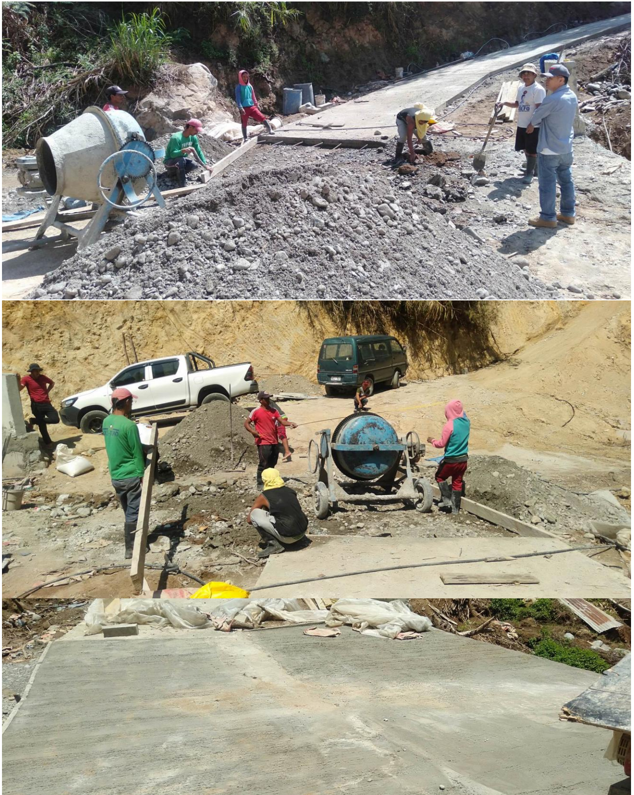
Photo 16. Colong-Sayangan Pavement Project.
