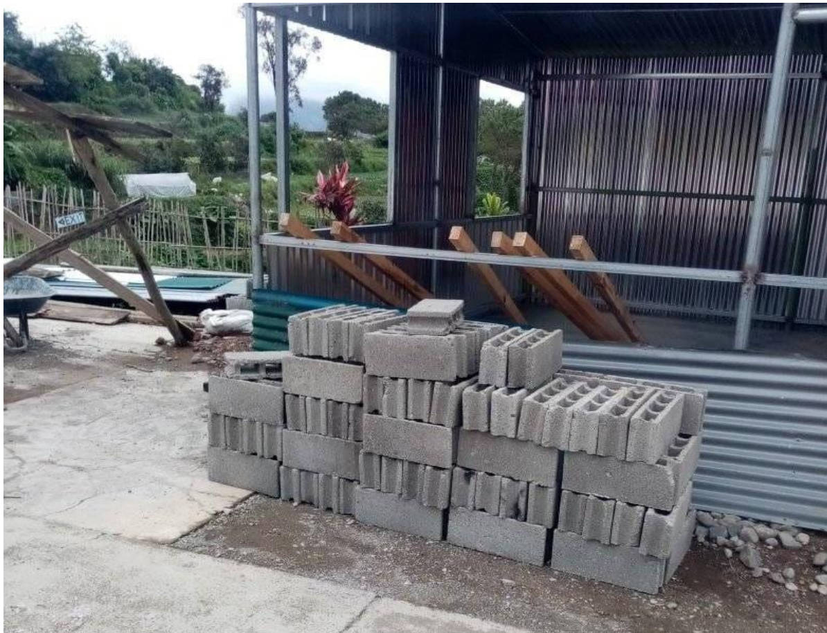
Photo 11. Hollow blocks and cement delivered to Lap-angan Suyoc/Palasa-an last Oct 03
