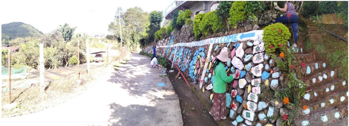
Photo 2. Repainting of the retaining wall of the CMDC office.
