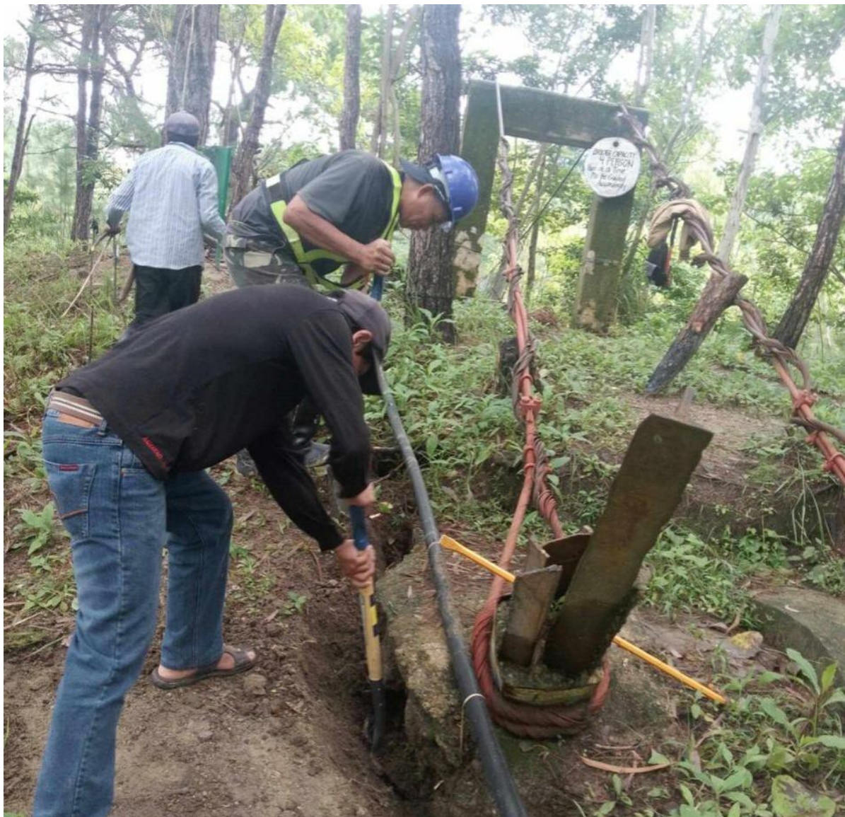
Photo 16. Donation of cement and gravel for the repairs of Petwagay Bridge.
