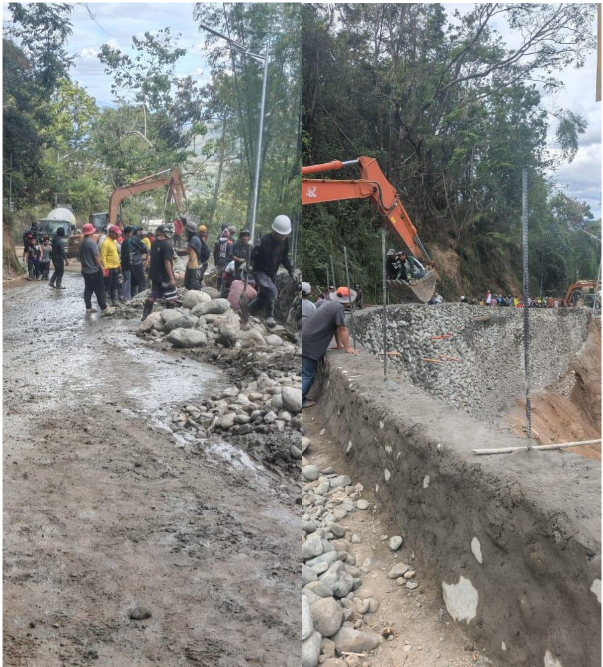
Photo 13. Road rehabilitation along Sitio Busan.
